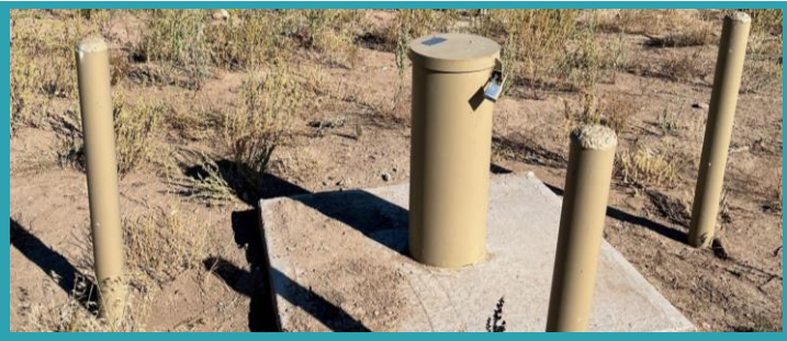
Photo: Water monitoring well
