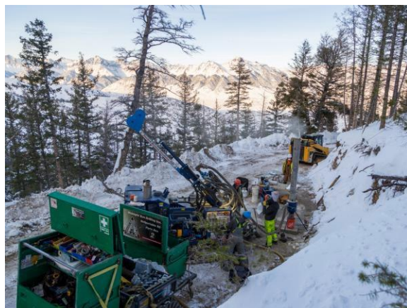
Photos: 2022 Red Star Drilling Program
